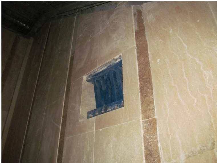
Figure ۱ - ۷ story steel structure in Karaj. TADAS dampers are installed in this project.
