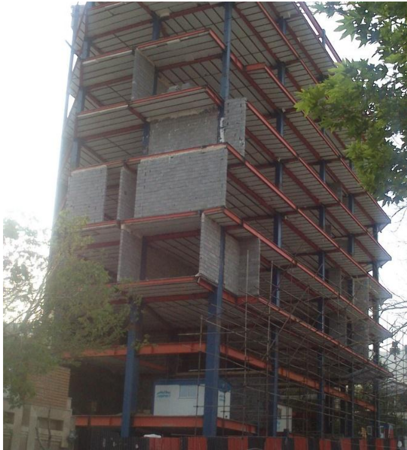
Figure ۲- ۱۳ Story steel structure in Tehran. TADAS dampers are used in this project
