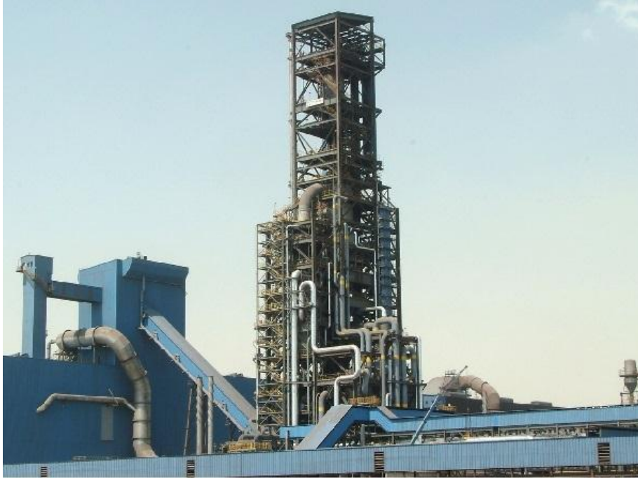
Figure ۴ - Gol -e- Gohar steel furnace in Sirjan with ۱۱۰ m height using viscous and TADAS dampers.
