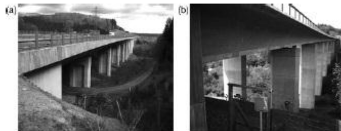
(a) Rümmecke Bridge and (b) Berbke Bridge
