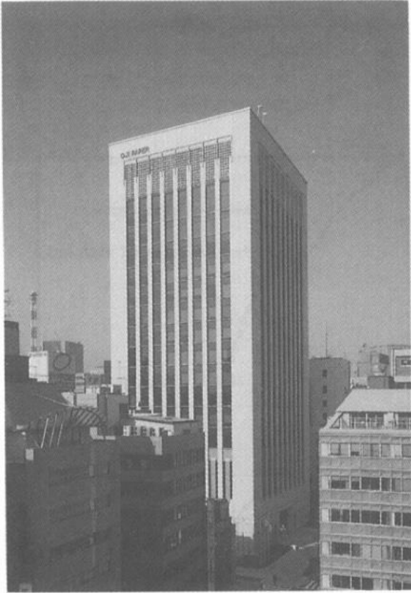
Ohji Corp. building (O building).
