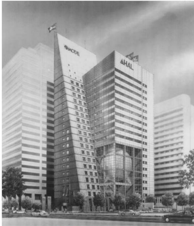
Perspective view of the building. Description of the building Name: School building of the Osaka Mode Fashion Institute Gakuen and the HAL Institute of Computer Technology . Use: Professional school Designer: Kajima Corporation. Total floor area: 31 800 m 2 . Building area: 2325 m 2 . Number of stories: 21 floors above ground, 3 basement floors, 2-story penthouse. Height: 75.54 m. Maximum height: 100.3 m
