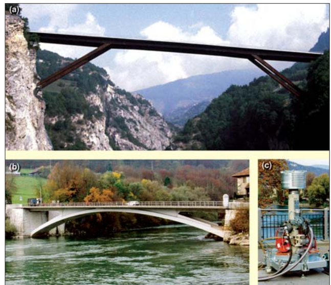
Figure 7. (a) Dala bridge; (b) Aarburg bridge; (c) electro-hydraulic vibrator used at Aarburg bridge.
