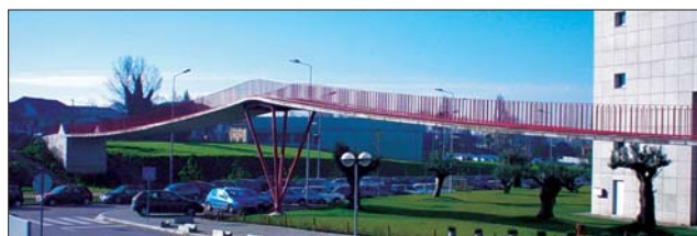
Figure 21. Stress-ribbon footbridge at FEUP Campus.
